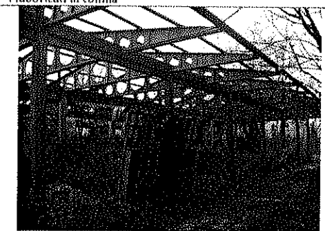
I fabbricati in collina
