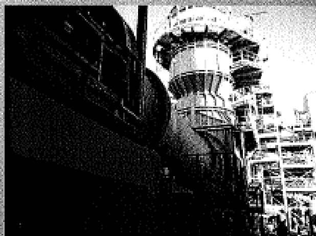
Incinerating line for Hospital waste with Kiln \varnothing 3,5 x 15 m - Bordeaux / France
