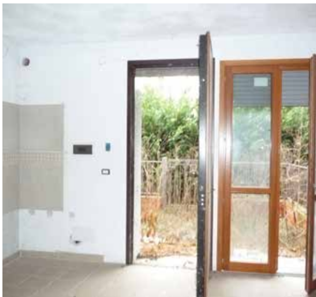
Locale cantina / piano "interrato"
