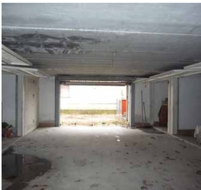
Vista corsie garages
