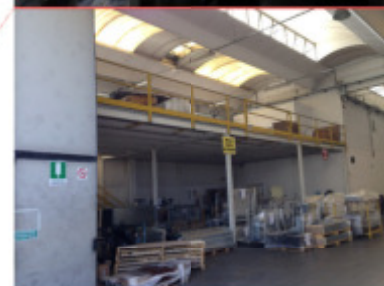
(4) area soppalcata abusiva
