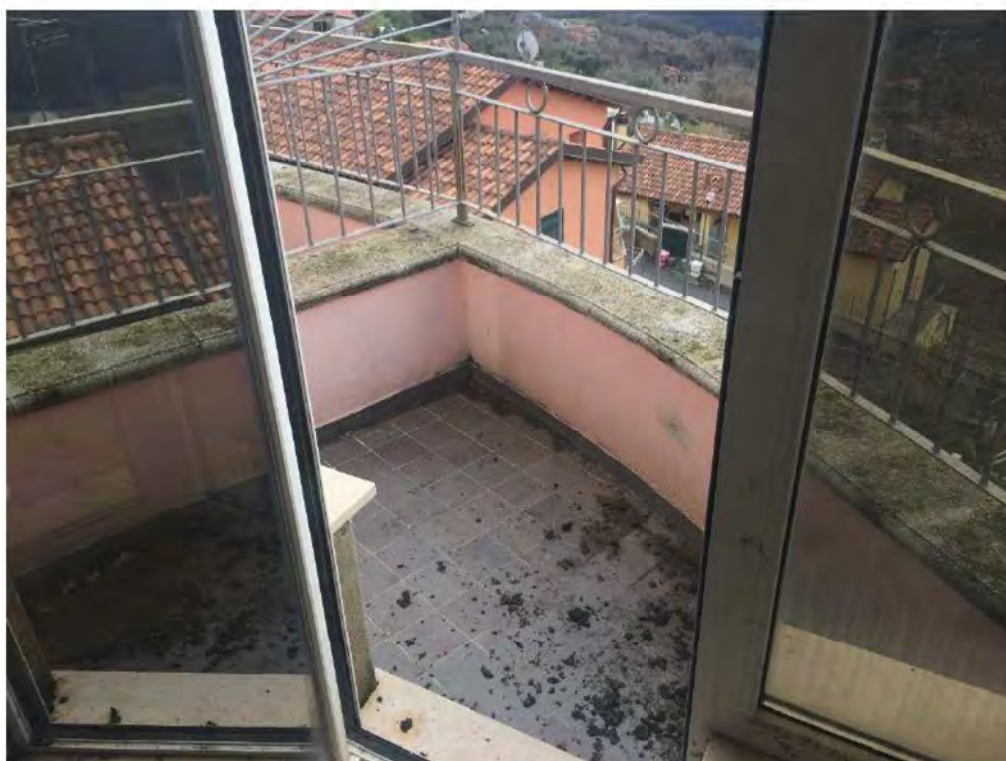
FOTO 10: PIANO TERRA BALCONE CAMERA
