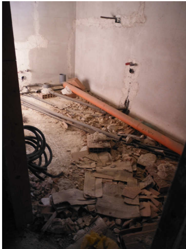
bagno piano interrato
