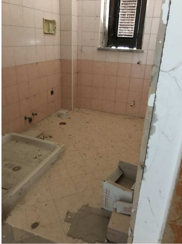
bagno piano terra
